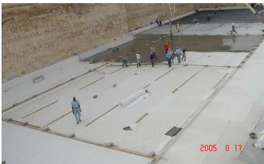
Installation of Water Stops and Execution of Protective Concrete
