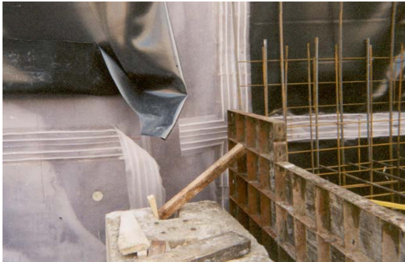
Dangers of mechanical impact to Waterproofing system
