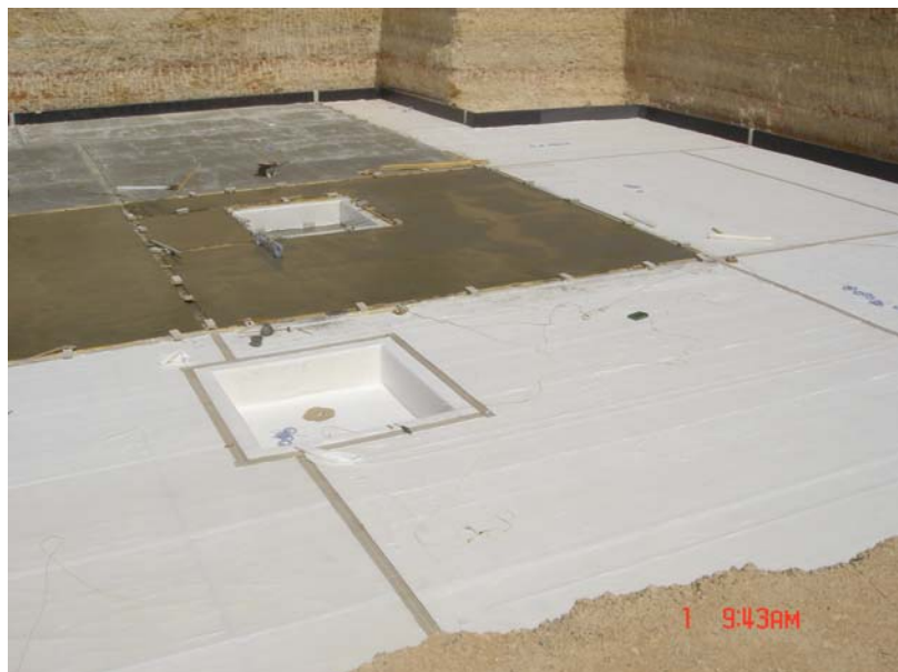
Execution of Protective Concrete
